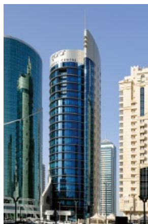
Doha, Qatar Financial Centre
