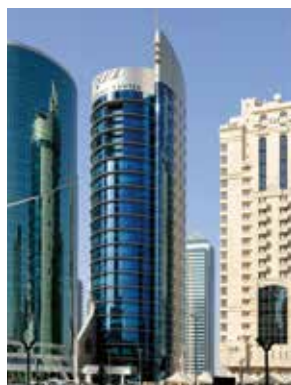
Doha, Qatar Financial Centre
